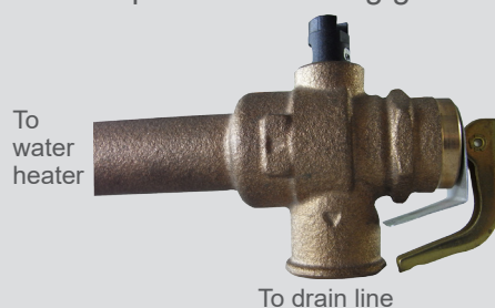
How to operate the easing gear
