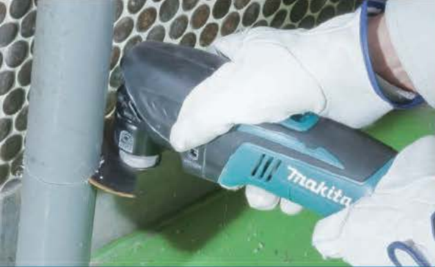
Cutting PVC, FRP pipes
