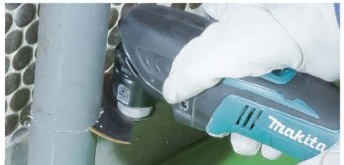
Cutting PVC, FRP pipes
