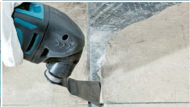
Scraping floor tiles
