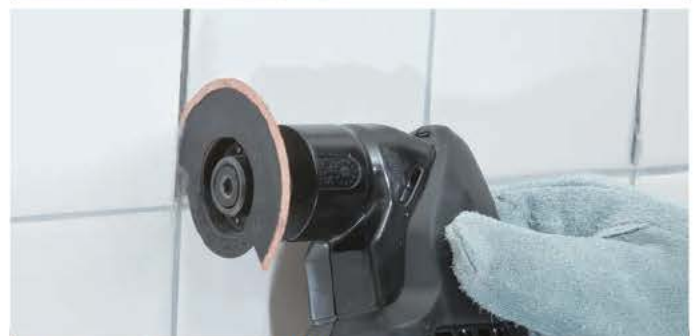
Routing joints on wall tiles (1) B-21490 (2) B-21509 (3) B-21521
