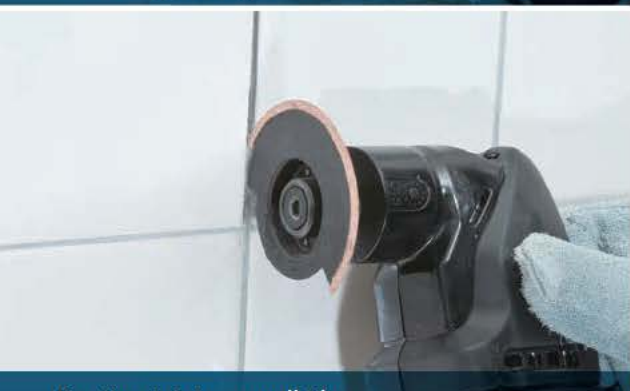
Routing joints on wall tiles
