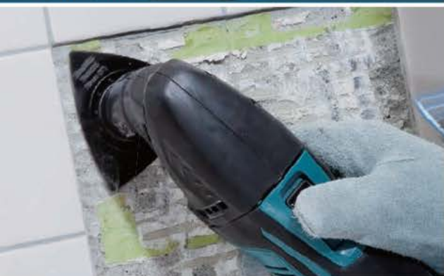
Removing mortar, tile adhesive
