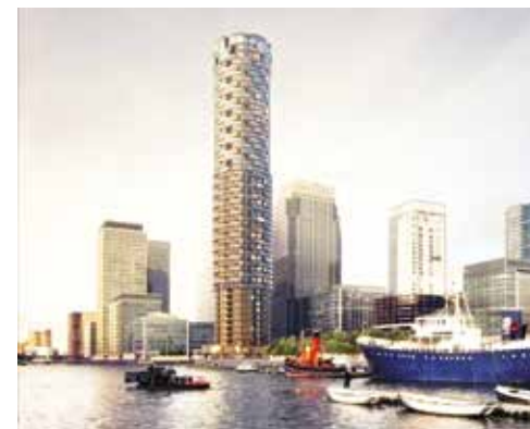
Wood Wharf, Canary Wharf, London, United Kingdom
