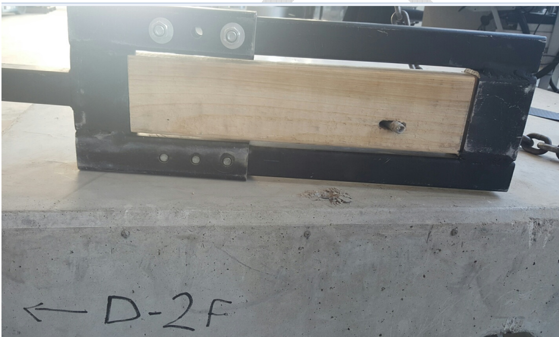
Figure 17: Anchor in shear failure
