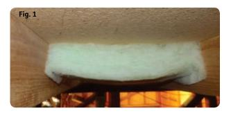
**Tight with no air gaps:** GreenStuf® Underfloor should be pulled tight between the joists to ensure there is no air-gap or air movement between the insulation material and the floor.
