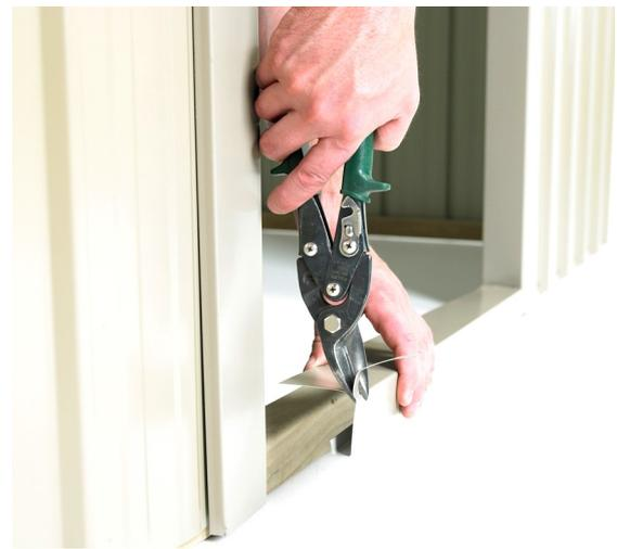
**Step2:** Measure and cut Doorstep Flashing (106) to fit in between Door Jamb. Position the Doorstep Flashing in between Door Jamb at bottom of doorway, nail through top of flashing using three 30mm Clouts. Repeat with the Overdoor Flashing (105).
