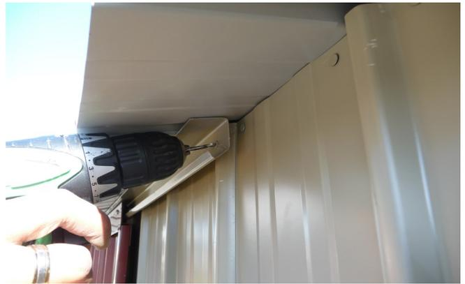
**Step 2:** Hang door in Door Track. At the right hand end of Door Track, adjust up or down so that the Door hangs parallel with shed. Fit one rivet at right hand end to hold in place. Repeat with left hand end of track.
