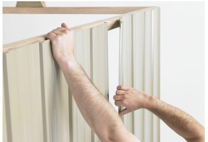
**Step 3: End Walls:** Lean Gable Wall Sheets against the shed to form gable shape. With the LIP flush with side of Stud tack in place ensuring the bottom of the Wall Sheet is 10mm above the bottom of the Bottom Plate. Tack on remaining Wall Sheets. Repeat with other gable end. If fitting a window, nail in Window Studs and Nog now. Refer to Window instructions.
