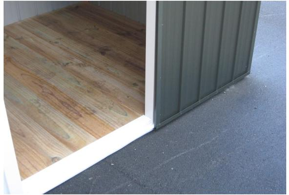
**Step 3:** Re-position Floor Board. Lay out remaining Floor Boards checking around Studs as you go. The last Floor Board may have to be cut to size.
