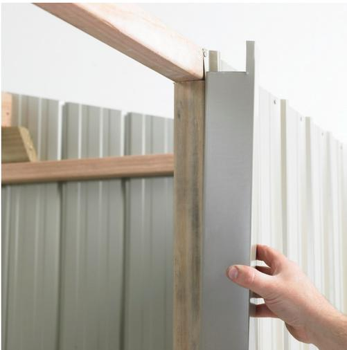
**Step1:** Fit Door Jamb Flashing (104) in between Top and Bottom Plates and hard against Stud. Attach Door Jamb Flashing with three rivets into Rib on the outside and three 30mm clouts into studs on the inside. Repeat with the other Door Jamb.
