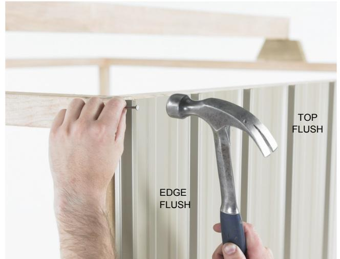
**Step 2: Back Wall:** Start at the right hand side. Position the first Wall Sheet with the LIP on the right hand side. Ensuring the LIP is flush with the side of the Studs and the top of the Wall Sheet is flush with the top of the Top Plate, tack in place. Position the next Wall Sheet with the LIP on the right hand side. Overlap as shown in (fig 1). Ensuring Wall Sheet is flush with top of Top Plate, tack in place. Repeat with remaining sheets.
