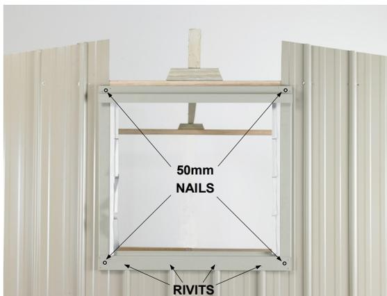
**Step 3:** Nail wall Sheets to window framing using 30mm clouts. (return to step 4 on page 7 and complete). Then fit Window Frame). Position Window Frame centrally on window opening and rivet it to ribs. Pre-drill holes in each corner and nail Window Frame to framing, using 50mm nails.
