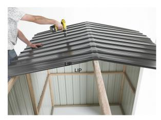
Step 3: Starting from the left hand end, centralize Roof on Ridge Beam. Ensure Roof is tight against end Wall Sheets, predrill then nail one 50mm Clout through Rib into the Ridge Beam. At the back, line up Ribs on the Roof Sheet with the Ribs on Wall Sheet. Using one 50mm Clout, nail through Rib into Back Top Plate. Repeat at the front.
