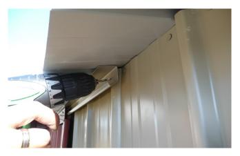
Step 2: Hang door in Door Track. At the right hand end of Door Track, adjust up or down so that the Door hangs parallel with shed. Fit one rivet at right hand end to hold in place. Repeat with left hand end of track.
