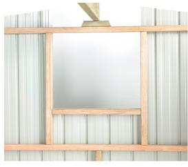
Step 2: On the inside of the shed, position studs and Nog centrally on window opening. Make sure the studs are parallel and nail into Top Plate and End Wall Nog.
