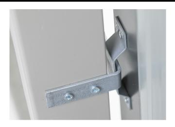
Step 2: Once door is hung, position the Locking Stays so they slide into the Locking Brackets easily. Screw Locking Stays to Door Jamb.
