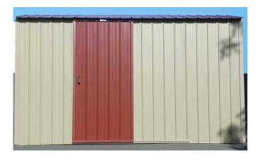
Step 3: Remove Door. Pre-drill holes into each Rib and at similar spacings into Over Door Flashing. At approximately 1/3 in from each end of Door Track put a 50mm nail. Fix rivets to rest of holes
