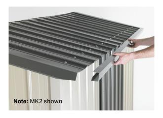
**Step 1:** Position Barge Flashing (102) on gable ends. Position a Spouting (A103) and rivet to the Barge Flashing at each end. Repeat with other Spouting.
