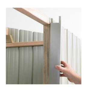
Step1: Fit Door Jamb Flashing (104) in between Top and Bottom Plates and hard against Stud. Attach Door Jamb Flashing with three rivets into Rib on the outside and three 30mm clouts into studs on the inside. Repeat with the other Door Jamb.
