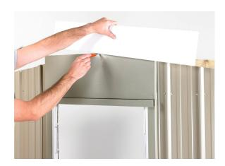
**Step 4:** If the Window is in the gable end, temporarily position the Over Panel above Window Frame. Following the same angle as the gable, mark and cut to suit.
