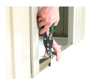
**Step2:** Measure and cut Doorstep Flashing (106) to fit in between Door Jambs. Position the Doorstep Flashing in between Door Jambs at bottom of doorway, nail through top of flashing using three 30mm Clouts. Repeat with the Overdoor Flashing (105).
