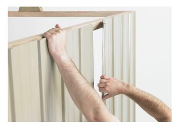
Step 3: End Walls: Lean Gable Wall Sheets against the shed to form gable shape. With the LIP flush with side of Stud tack in place ensuring the bottom of the Wall Sheet is 10mm above the bottom of the Bottom Plate. Tack on remaining Wall Sheets. Repeat with other gable end. If fitting a window, nail in Window Studs and Nog now. Refer to Window instructions.
