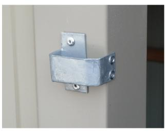
Step 3 On the left hand Door Jamb, position latch so that the hook on the door handle will be secure and go in and out easily. Rivet in place with four rivets.
