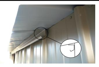
Step 1: Position Door Track (107) on front wall up against underside of Roof, with left hand end flush with the left side of the left hand Door Jamb Flashing. Predrill hole in centre and rivet in place. Remove ALL drill filings
