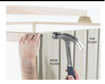
Step 2: Back Wall: Start at the right hand side. Position the first Wall Sheet with the LIP on the right hand side. Ensuring the LIP is flush with the side of the Studs and the top of the Wall Sheet is flush with the top of the Top Plate, tack in place. Position the next Wall Sheet with the LIP on the right hand side. Overlap as shown in (fig 1). Ensuring Wall Sheet is flush with top of Top Plate, tack in place. Repeat with remaining sheets.
