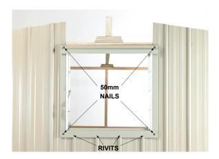
Step 3: Nail wall Sheets to window framing using 30mm clouts. (return to step 4 on page 7 and complete). Then fit Window Frame). Position Window Frame centrally on window opening and rivet it to ribs. Pre-drill holes in each corner and nail Window Frame to framing, using 50mm nails.
