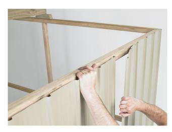
Step 3: End Walls: Lean Gable Wall Sheets against the shed to form gable shape. With the LIP flush with side of Stud tack in place ensuring the bottom of the Wall Sheet is 10mm above the bottom of the Bottom Plate. Tack on remaining Wall Sheets. Repeat with other gable end. If fitting a window, nail in Window Studs and Nog now. Refer to Window instructions.
