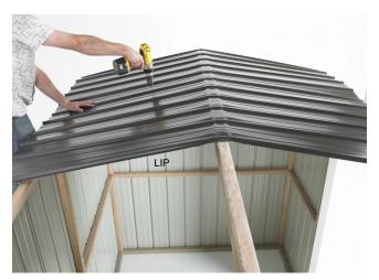
Step 1: Position first Roof Sheet centrally over Ridge Beam on the right hand end of shed with the LIP on the left hand side. (For sheds with a Clear Roof Panel, go to the next page). Position the next Roof Sheet. Ensure it overlaps correctly then rivet together, one rivet in the centre and one 600mm and 1200mm down from the centre on both sides. Fit remaining Roof Sheet.
