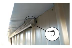
Step 3: Hang left hand door in Door Track. At the left hand end of Door Track, adjust up or down so that the Door hangs parallel with shed. Fit one rivet at left hand end to hold in place.
