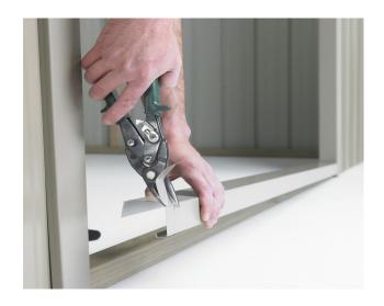
**Step2:** Measure and cut Doorstep Flashing (A106) to fit in between Door Jambs. Positioning the Doorstep Flashing in between Door Jambs at bottom of doorway, nail through top of flashing using five 30mm Clouts. Repeat with the Overdoor Flashing (A105).
