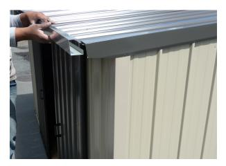
Step 1: Attach left hand and right hand barges (C102 & D102) together with three rivets at top overlap. Position Barge Flashings on gable ends. Position Spouting (C103)on the shed and rivet to barge Flashing at each end. Repeat with other Spouting.
