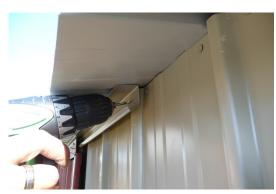
Step 5: Clean out ALL drill filings. Also make sure the Wheels are cleaned of drill filings. Rehang Doors, then insert door stops into the pre drilled holes at end of tracks as shown in diagram. Tighten with two spanners
