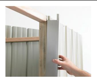
Step1: Fit Door Jamb Flashing (A104) in between Top and Bottom Plates and hard against Stud. Attach Door Jamb Flashing with three 30mm clouts into studs on the inside and three rivets into Rib on the outside. Pre-drill holes on the outside to protect flashing. Repeat with the other Door Jamb.
