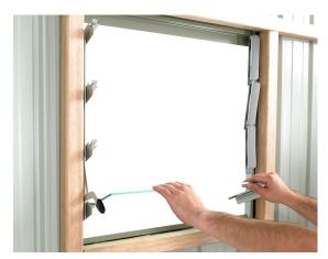
**Step 6:** From the inside of the shed, slide Louvre Glass into Louvre Units attached to the Window Frame. Bend up tabs to keep Glass in position.
