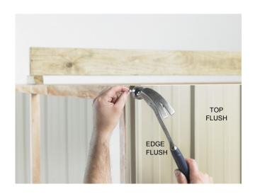
Step 2: Back Wall: Position the first Wall Sheet with the LIP on the right hand side. Ensuring the LIP is flush with the side of the Stud and the top of the Wall Sheet is flush with the top of the Top Plate, tack in place. Position the next Wall Sheet with the LIP on the right hand side. Overlap as shown in fig.1 (page 7). Ensuring Wall Sheet is flush with top of Top Plate, tack in place. Repeat with remaining two sheets.
