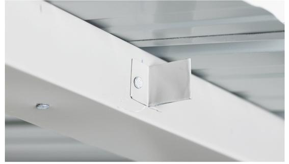
**Step 2:** Position right hand Door Track (D107) on front wall up against underside of Roof, with left hand end hard against the Centre Door Stop. Pre-drill hole in centre and rivet in place. Remove ALL drill filings
