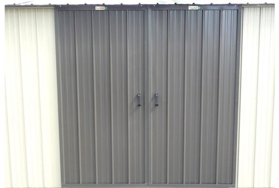
**Step 4:** Position left hand Door Track (C107). Follow Steps 2 and 3 to hang left hand Door. Where Door Tracks meet in the centre, adjust up and down so that the Doors parallel, then rivet in place. Remove Doors. Pre-drill holes into each Rib and at similar spacings into Overdoor Flashing. At approximately 1/3 in from each end of Door Tracks put a 50mm nail. Rivet rest of holes.
