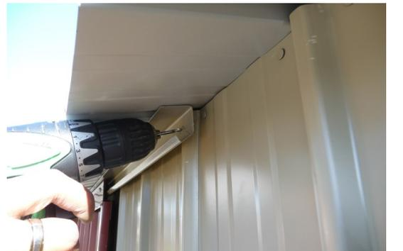
**Step 5:** Clean out ALL drill filings. Also make sure the Wheels are cleaned of drill filings. Re-hang Doors, then insert door stops into the pre drilled holes at end of tracks as shown in diagram. Tighten with two spanners
