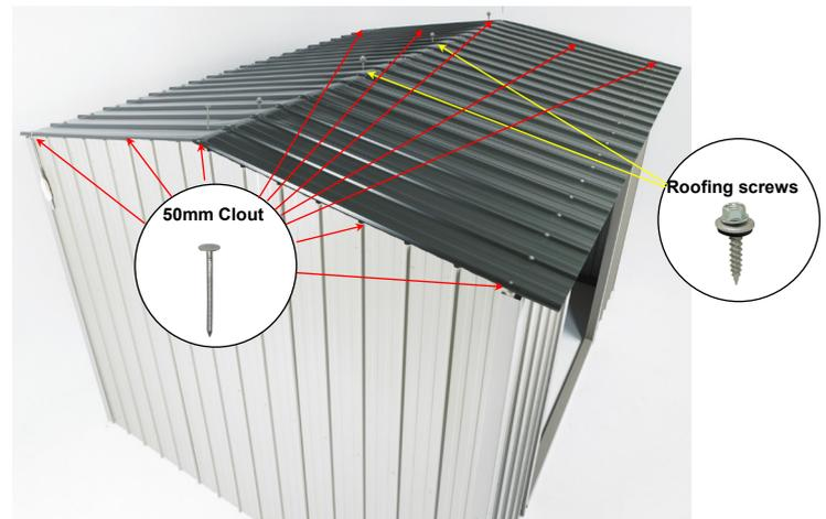
**Step 2:** Starting from the left hand end, centralize Roof on Ridge Beam. Ensure Roof is tight against end Wall Sheets, predrill then nail one 50mm Clout through Rib into the Ridge Beam. At the back, line up Ribs on the Roof Sheet with the Ribs on Wall Sheet. Using one 50mm Clout, nail through Rib into Back Top Plate. Repeat at the front.
