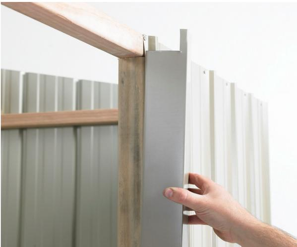
**Step1:** Fit Door Jamb Flashing (A104) in between Top and Bottom Plates and hard against Stud. Attach Door Jamb Flashing with three 30mm clouts into studs on the inside and three rivets into Rib on the outside. Pre-drill holes on the outside to protect flashing. Repeat with the other Door Jamb.
