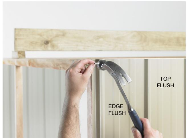
**Step 2: Back Wall:** Position the first Wall Sheet with the LIP on the right hand side. Ensuring the LIP is flush with the side of the Stud and the top of the Wall Sheet is flush with the top of the Top Plate, tack in place. Position the next Wall Sheet with the LIP on the right hand side. Overlap as shown in *fig.1* (page 7). Ensuring Wall Sheet is flush with top of Top Plate, tack in place. Repeat with remaining two sheets.
