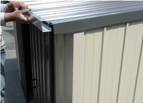
**Step 1:** Attach left hand and right hand barges (C102 & D102) together with three rivets at top overlap. Position Barge Flashings on gable ends. Position Spouting (C103) on the shed and rivet to barge Flashing at each end. Repeat with other Spouting.
