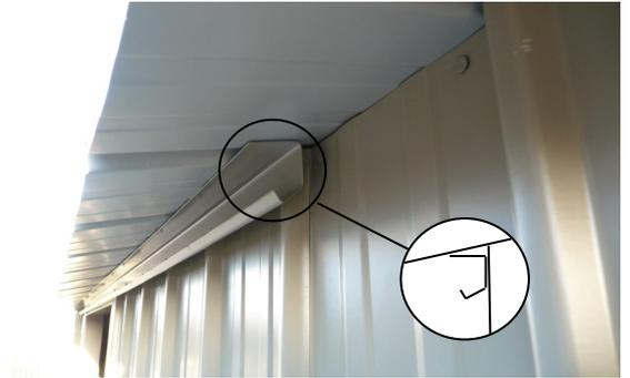
**Step 3:** Hang left hand door in Door Track. At the left hand end of Door Track, adjust up or down so that the Door hangs parallel with shed. Fit one rivet at left hand end to hold in place.
