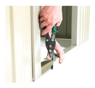
**Step2:** Measure and cut Doorstep Flashing (106) to fit in between Door Jambs. Position the Doorstep Flashing in between the Door Jambs at bottom of doorway, nail through top of flashing using five 30mm Clouts. Repeat with the Overdoor Flashing (105).
