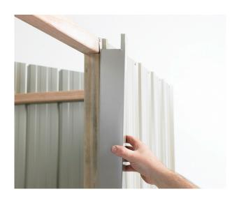
**Step1:** Fit Door Jamb Flashing (104) in between Top and Bottom Plates and hard against Stud. Attach Door Jamb Flashing with three rivets into Rib on the outside and three 30mm clouts into studs on the inside. Repeat with the other Door Jamb.
