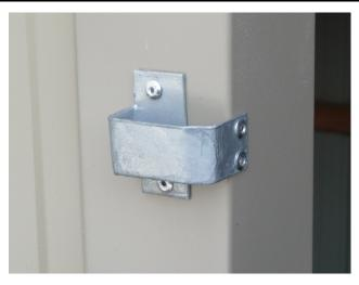
Step 3 On the left hand Door Jamb, position latch so that the hook on the door handle will be secure and go in and out easily. Rivet in place with four rivets.
