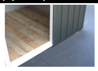
Step 4: Nail in each Floor Board, two 50mm nails in each end and two into Joists. Measure and cut Floor Flashing (110) to fit in between Door Jamb Flashings and nail in place using 50mm Clouts.
