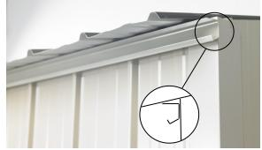
**Step 1:** Position Door Track (107) on front wall up against underside of Roof, with right hand end flush with the right hand corner. Pre-drill hole in centre and rivet in place. Remove ALL drill filings
