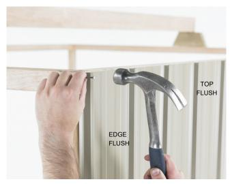
Step 2: Back Wall: Position the first Wall Sheet with the LIP on the right hand side. Ensuring the LIP is flush with the side of the Studs and the top of the Wall Sheet is flush with the top of the Top Plate, tack in place. Position the next Wall Sheet with the LIP on the right hand side. Overlap as shown in (fig 1). Ensuring Wall Sheet is flush with top of Top Plate, tack in place. Repeat with remaining sheet.
