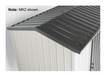
Step 2: Centralise Barge Flashing on gable end and rivet in place, one rivet into every second Rib.
